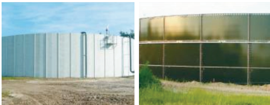
Figure 10.13 Concrete and steel tanks for liquid manure
