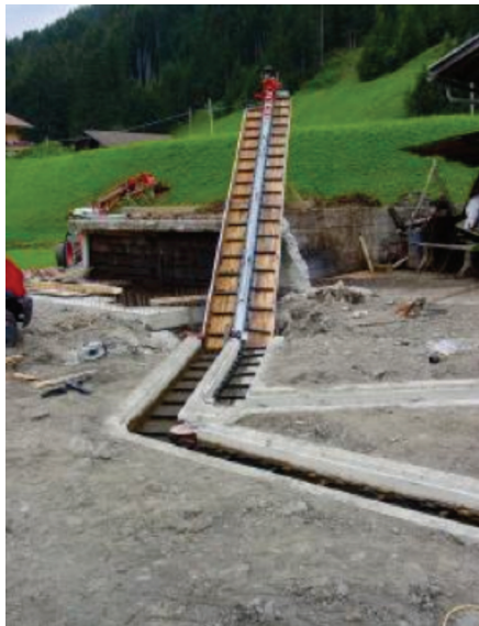
Figure 10.6 Removal mechanisms with chains [4]
